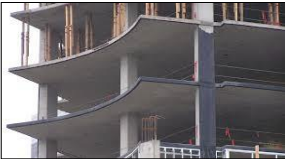
Figure 3: Reinforced concrete beam-supported slab system
