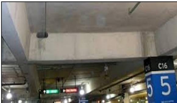
Figure 3: Reinforced concrete beam-supported slab system
